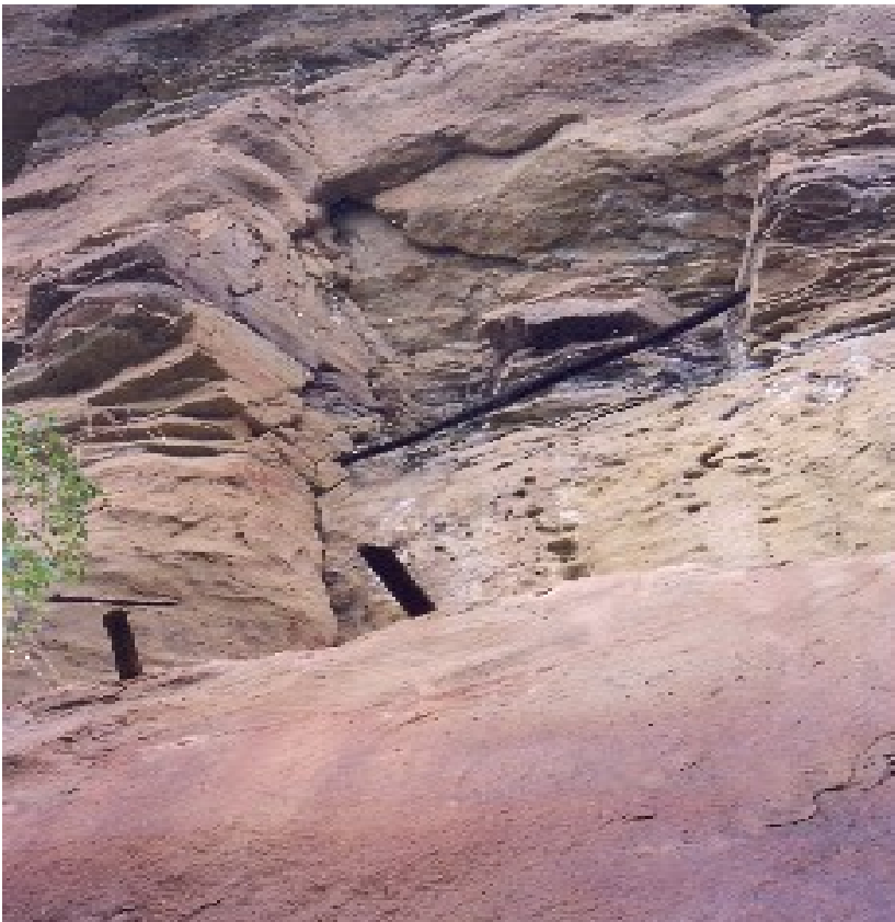
Figure 3.22: Poles extending from ledge identical to 1931 description, as observed in 2002 (J.D. Spangler).
