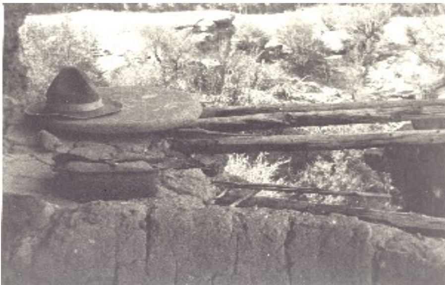
Figure 3.31: View of roof beams at 42Em741 as observed in 1931 (Peabody Museum U-31-79).
