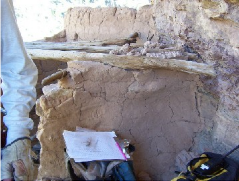
Figure 3.34: View of wall construction with vegetal binding, as observed in 2005 (K.R. Barlow, courtesy of National Geographic Society Committee for Research and Exploration).
