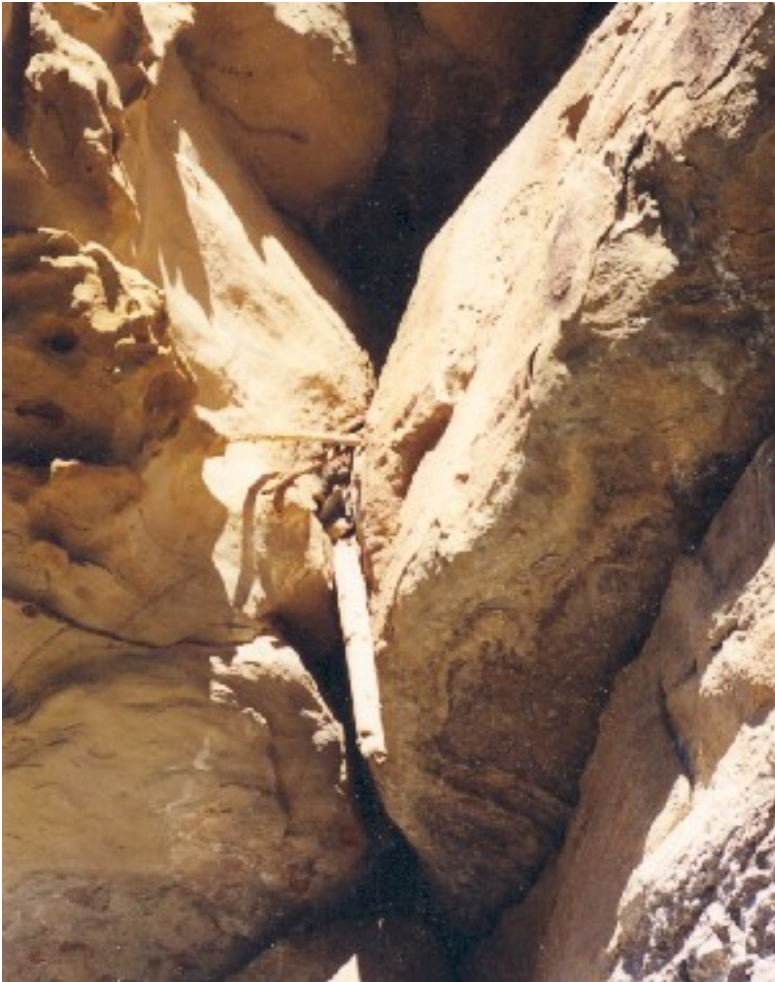
Figure 3.23: View of collapsed construction materials at 42Em3110, as observed in 2003 (J.D. Spangler)
