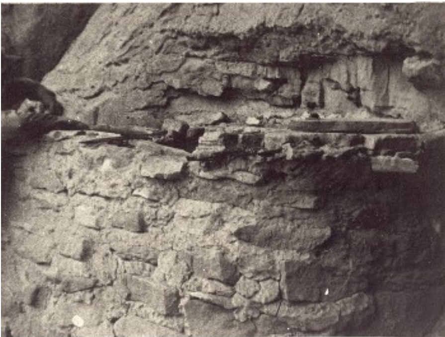
Figure 3.73: Exterior wall construction at 42Em761, as observed in 1931 (Peabody Museum U-31-84).
