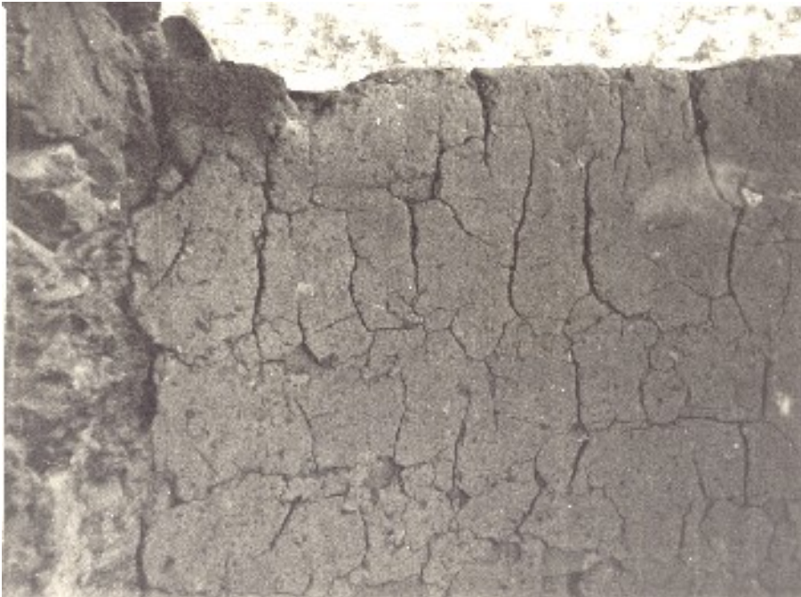
Figure 3.30: Close-up view of wall matrix at 42Em741, as observed in 1931 (Peabody Museum U-31-78).
