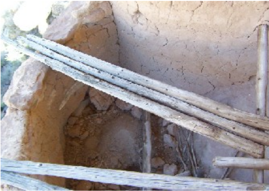
Figure 3.33: View of remnants of collapsed roof superstructure, as observed in 2005 (K.R. Barlow, courtesy of National Geographic Society Committee for Research and Exploration).
